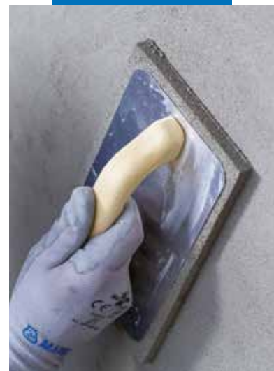
Floating the surface of Planitop Smooth & Repair R4
