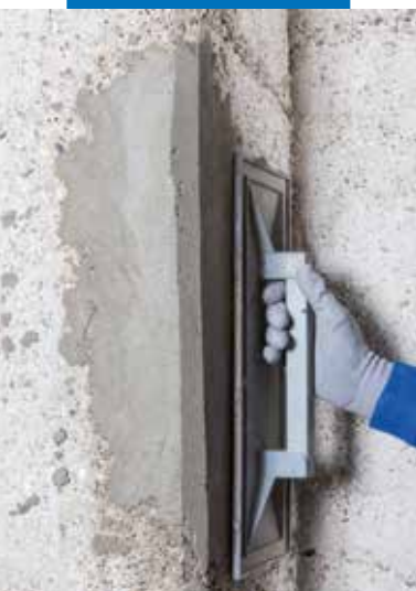
Floating the surface of Planitop Smooth & Repair R4 to create a smooth finish
