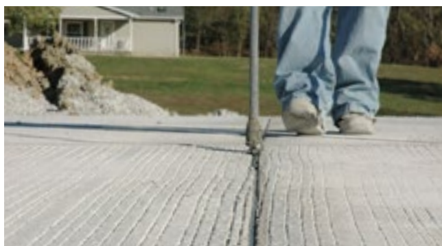
Installing DOWSIL™ 890-SL Silicone Joint Sealant
