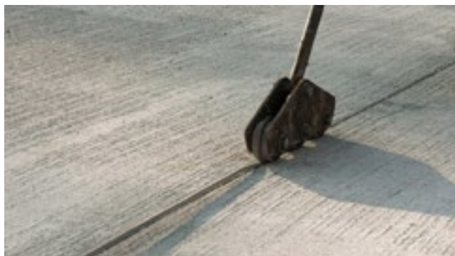
Installing the Backer Rod
