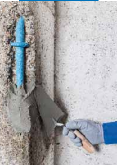
Applying Planitop Smooth & Repair R4 with a trowel
