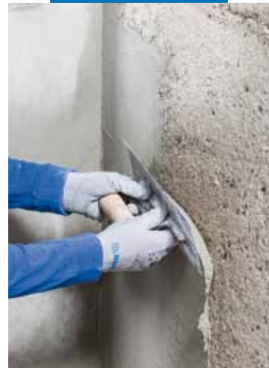
Applying Planitop Smooth & Repair R4 with a putty knife
