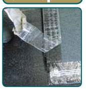
Unique factory-applied adhesive treatment at membrane overlaps for enhanced sealability.
